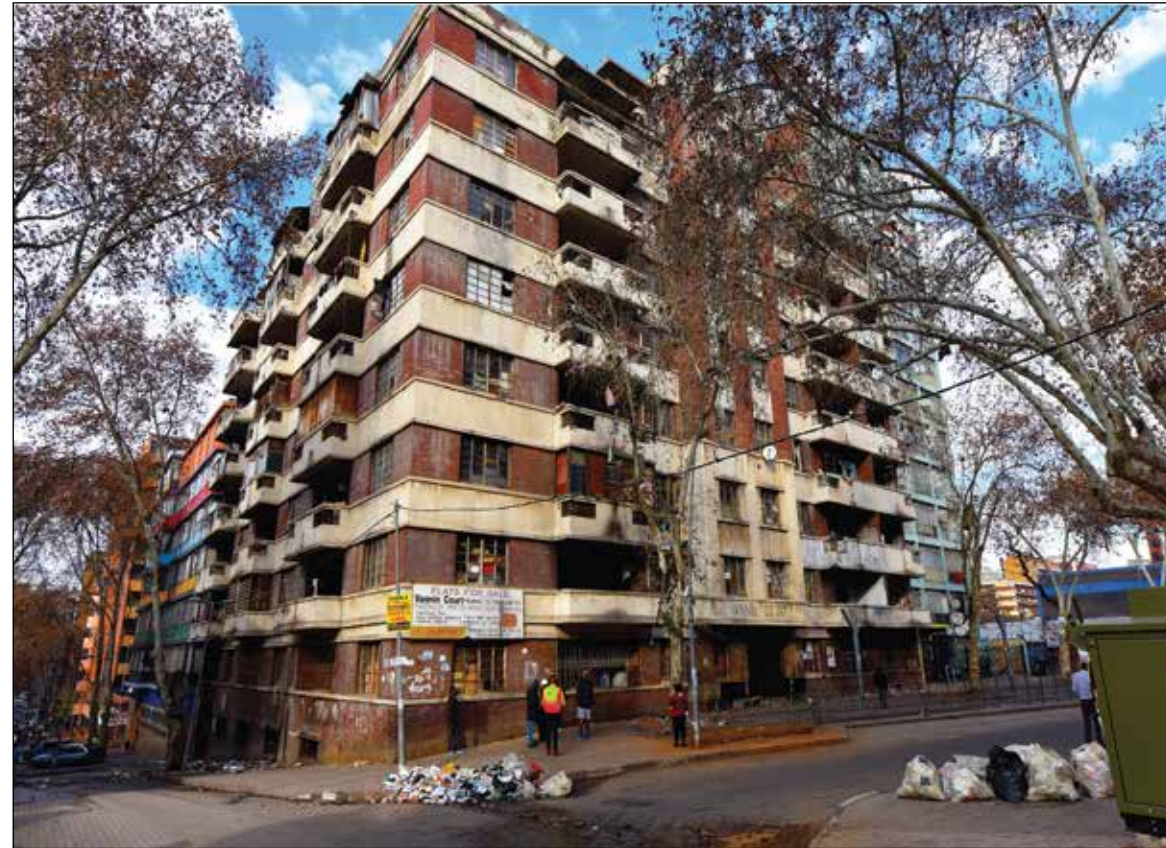
Urban blight: Musa Makhunga is determined to rid Joburg of buildings like this, where there is no water, no safety, and no services. Photo: Eddie Mtsweni
